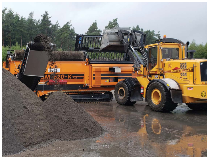
PFAS Soil being Immobilised with RemBind
