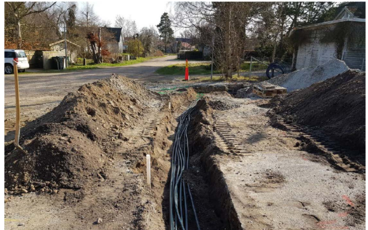
Excavation during Fire Station Expansion
